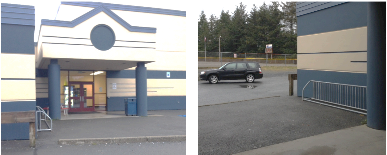
Figure 2: Pool Entrance to Blatchley and View from Pool Entrance Across Parking Lot to City Ball Field
